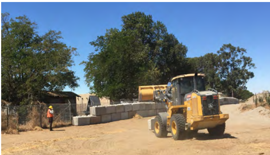
Refuge staff placing block on the Stamm Unit. Photo: FWS
