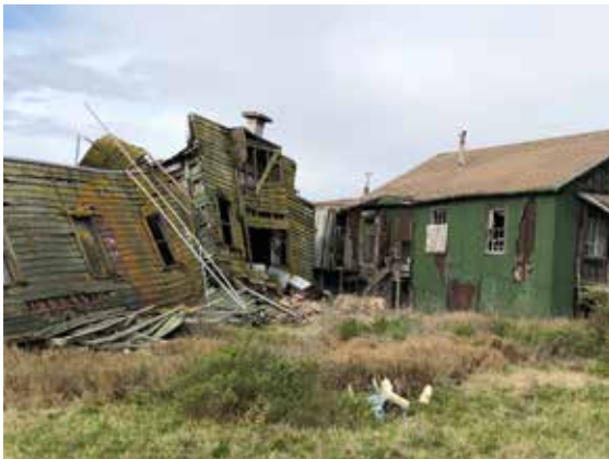
Decaying buildings: Former Detjen Duck Club, the newest addition to the refuge
